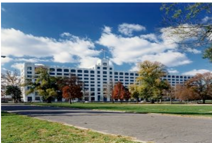
Baltimore’s Montgomery Ward warehouse - vacant for 20 years – was redeveloped due to creative local, state, and federal financing.
